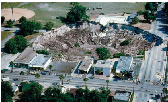
▲ Figure 17.17 Sinkhole formation. An underground void develops as limestone, \text{CaCO}_3(s) , dissolves. Collapse of the overlying ground into an underground cavity causes sinkhole formation. The large sinkhole shown here occurred in Orlando, Florida and destroyed several buildings and part of a highway.
